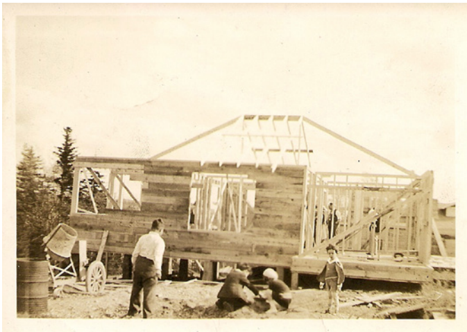
Elman cottage under construction in Pamdenec, early 1920s.
